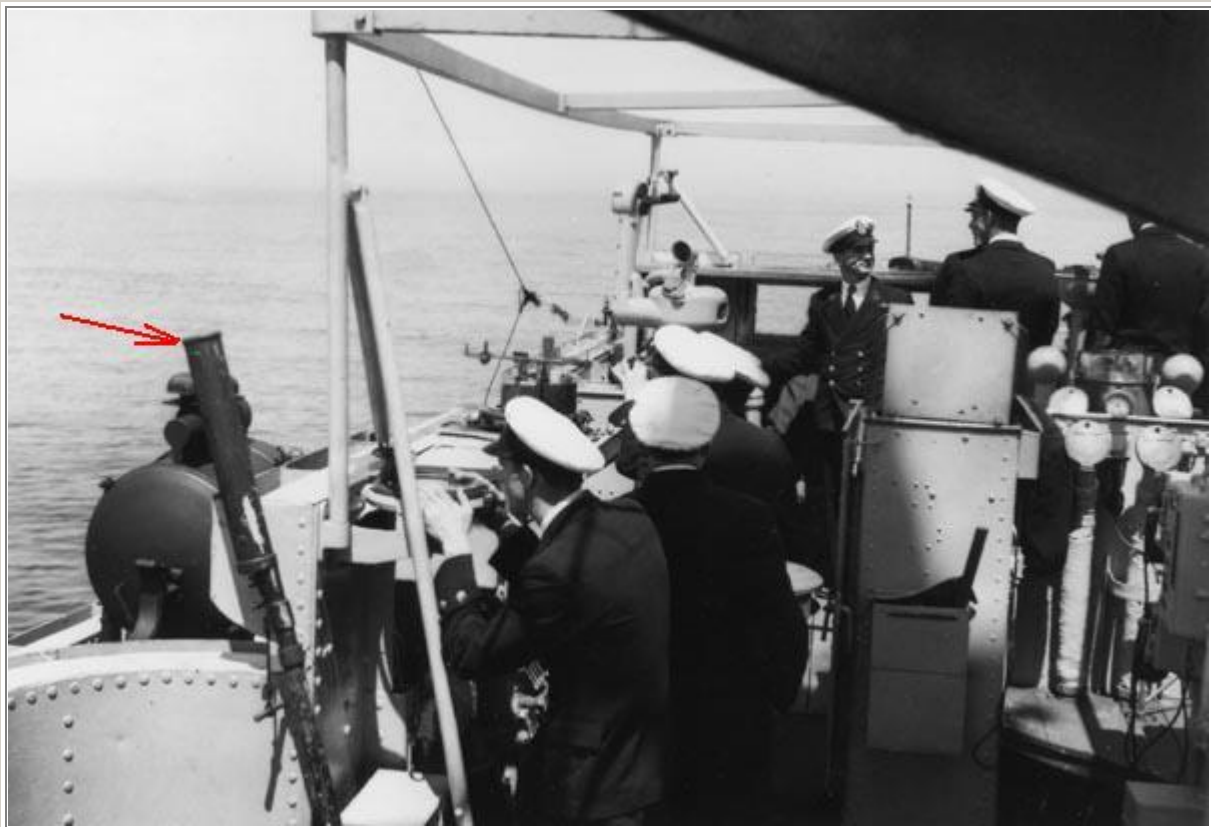
This photo, taken on the bridge of HMCS HAIDA in the late 1940's, shows the position of the port side Schermuly signal rocket launcher. Signal rockets would be fitted into the tubes when going to sea and stowed when in harbour. The rocket would only be fired in an emergency using a Copper Friction tube that was fitted in a small opening with a breech closing to keep it in place. This duty was normally performed by the Gunners Yeoman as opposed to a "bunting tosser" Yeoman. (Photo courtesy HMCS HAIDA Archives)
